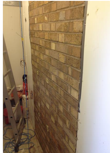
b) Solid brick wall (w/o insulation) completed
