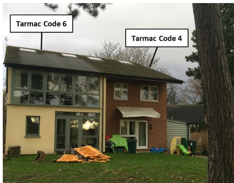
Figure 6-2: External view of the Tarmac Masonry Homes
