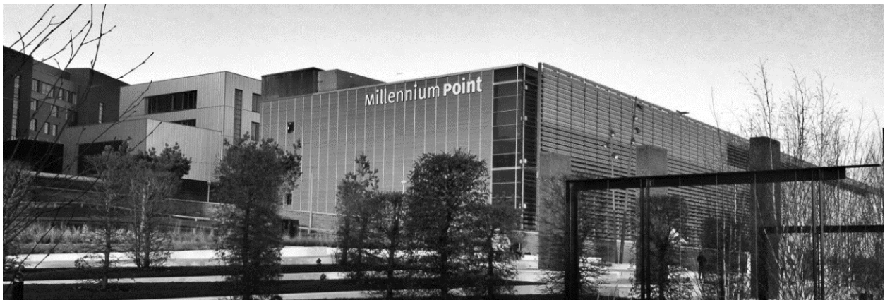
Fig. 7.3.1-3. Millennium Point, Birmingham designed by Nicholas Grimshaw & Partners
