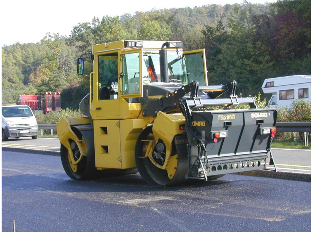
Figure 30: Gritting Operations for German SMA
