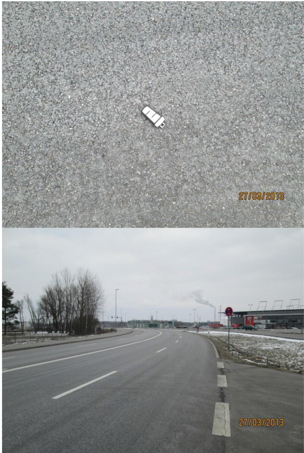
Figure 33: Ingolstadt / Audi Sportpark, SMA 11 S + SMA Binder 16
