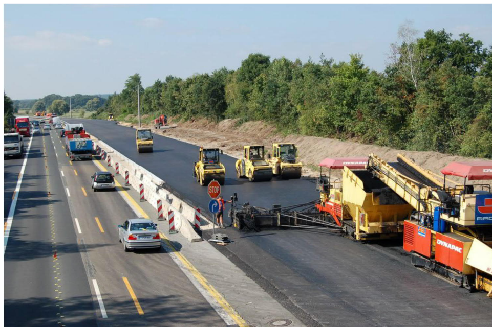
Figure 31: The Use of Wide Pavers, Multiple Roller Compactors under Full Closures
