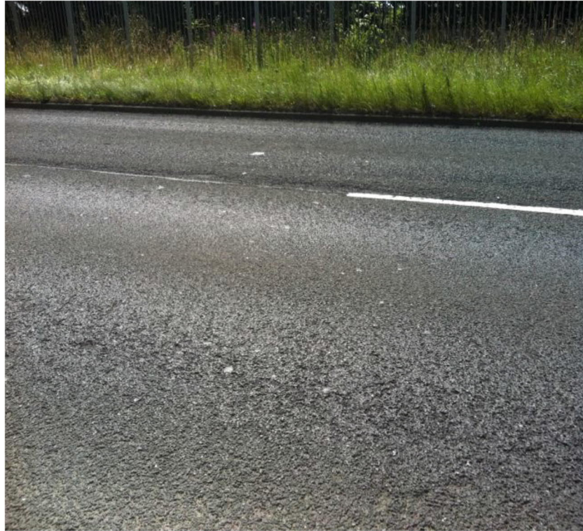
Figure 12: A19 Royal Quays - Site Photographs (Jones and Carswell, 2012)
