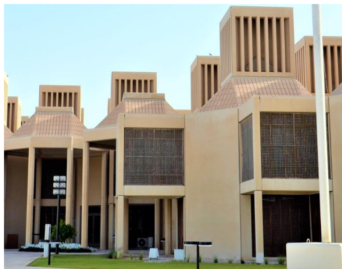
Figure 2-20b Modern wind catcher in Qatar University Doha, Qatar. Source; https://www.archnet.org/sites/288
