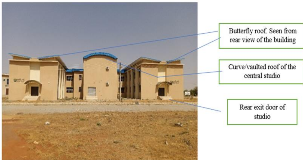
Figure 3-8 South Elevation of the Studio Complex showing structural roofing styles.
