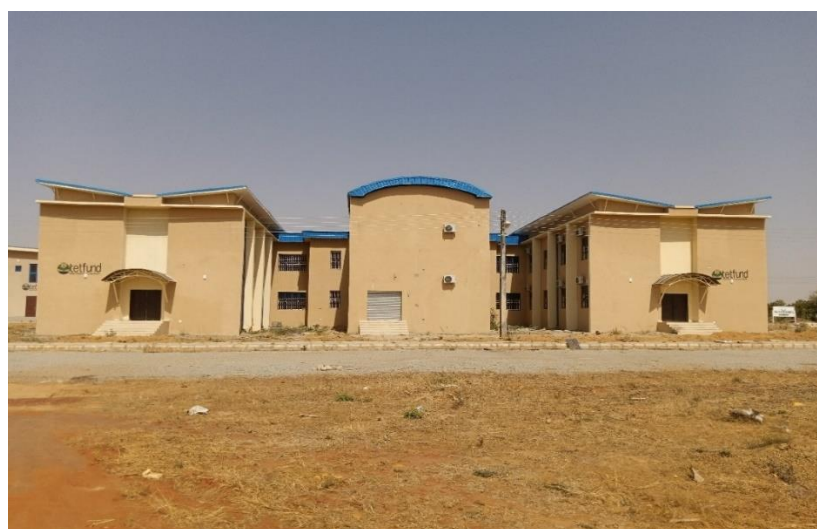
Figure 3-7 South Elevation of the Architectural Studios Complex.
